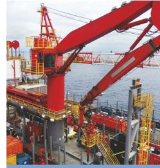
PLATFORM CRANES AND SHEAVES
